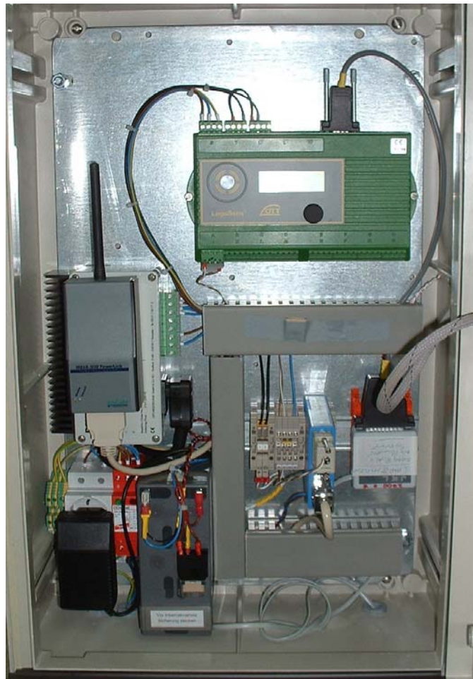
Cabinet containing the data logger
